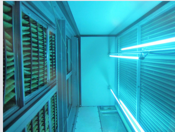
In-Duct/Coil UVGI
